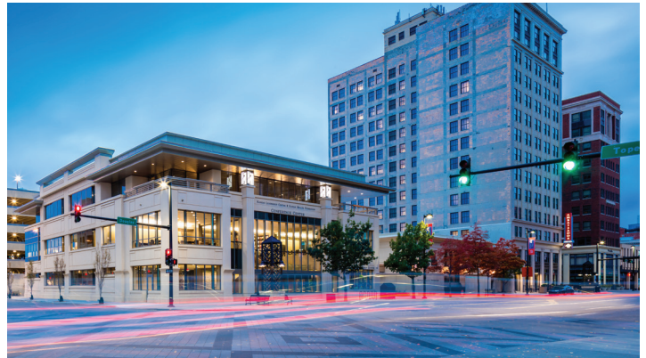
First new building on Douglas Avenue in 38 years, Kansas Leadership Center, is completed.
