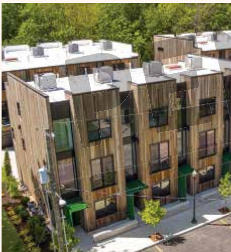
Trailhead Mews, Bentonville, AR
