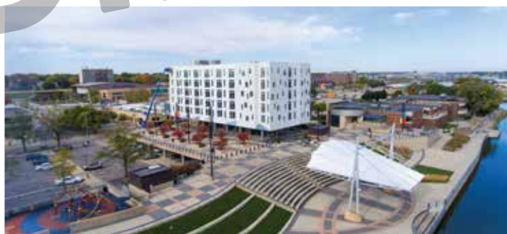
Art Bloc in Waterloo, Iowa is a 72-unit mixed-use riverfront development in downtown that overlooks an amphitheater and riverfront promenade.
