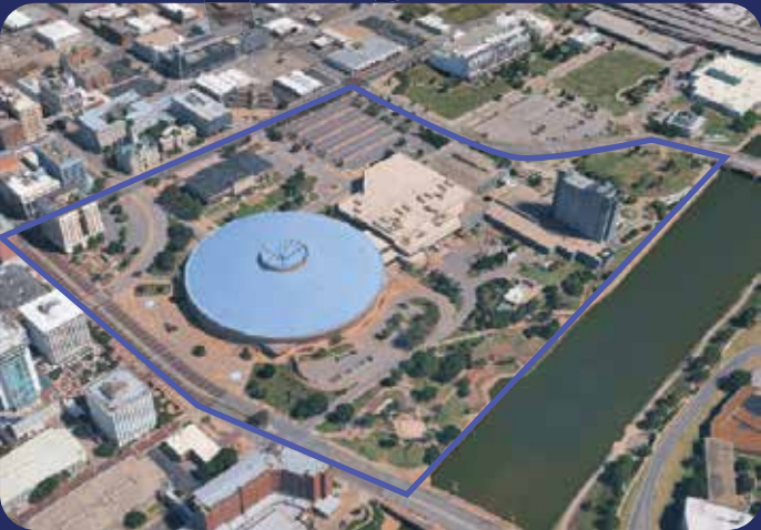
EXISTING CONDITION Convention Center, Century II
