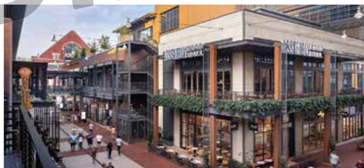
Fifth + Broadway in Nashville, Tennessee is a new mixed-use development on the site of the old Nashville Convention Center featuring shopping, a food hall, and office space.
