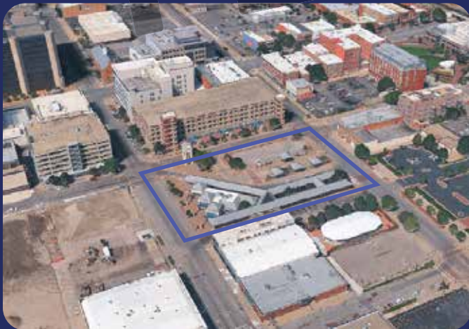
EXISTING CONDITION Wichita Transit Center
