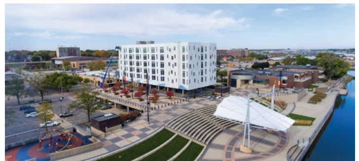
Art Bloc in Waterloo, Iowa is a 72-unit mixed-use riverfront development in downtown that overlooks an amphitheater and riverfront promenade.
