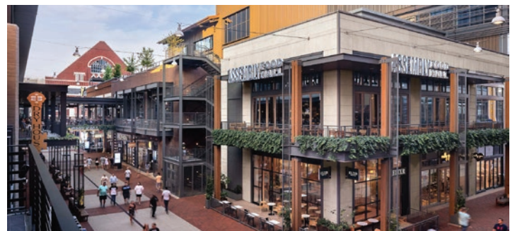
Fifth + Broadway in Nashville, Tennessee is a new mixed-use development on the site of the old Nashville Convention Center featuring shopping, a food hall, and office space.
