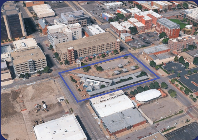
EXISTING CONDITION Wichita Transit Center
