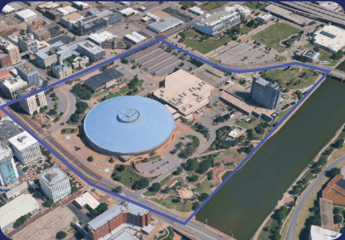
EXISTING CONDITION Convention Center, Century II
