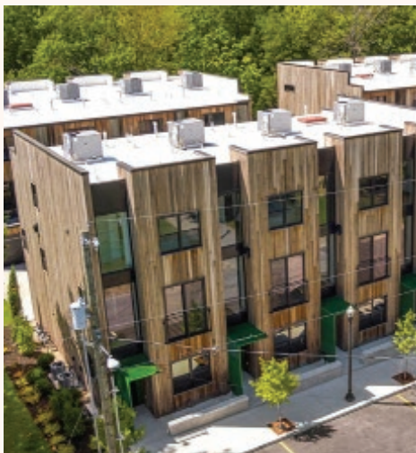
Trailhead Mews, Bentonville, AR
