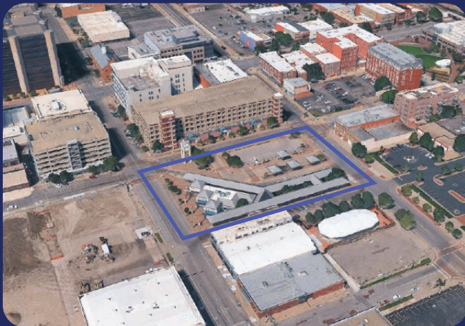
EXISTING CONDITION Wichita Transit Center
