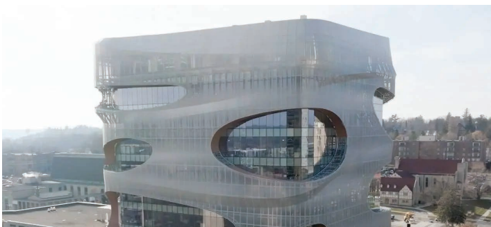
Mayo Clinic in Rochester, Minnesota is undergoing a $5 billion comprehensive redevelopment that unifies clinical, research, and patient care facilities into pedestrian-centered neighborhoods.
