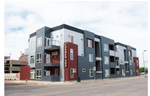
Corner 365 Apartments, Wichita, KS
