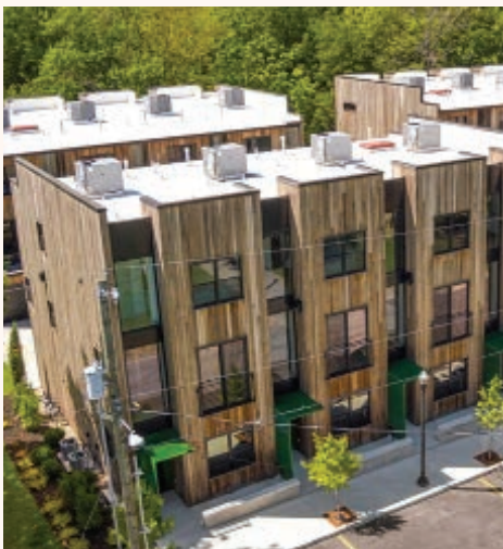
Trailhead Mews, Bentonville, AR
