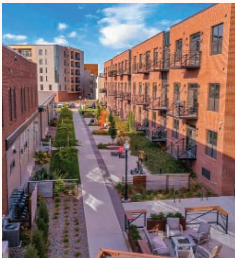
Railyard Flats, Sioux Falls, SD
