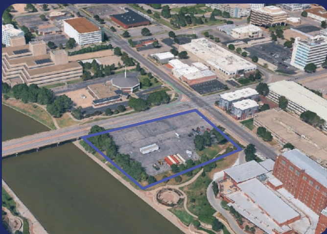
EXISTING CONDITION Surface Parking Lot
