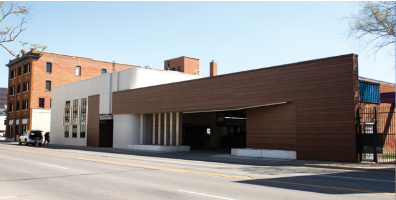
SPT Architecture Headquarters N/A
