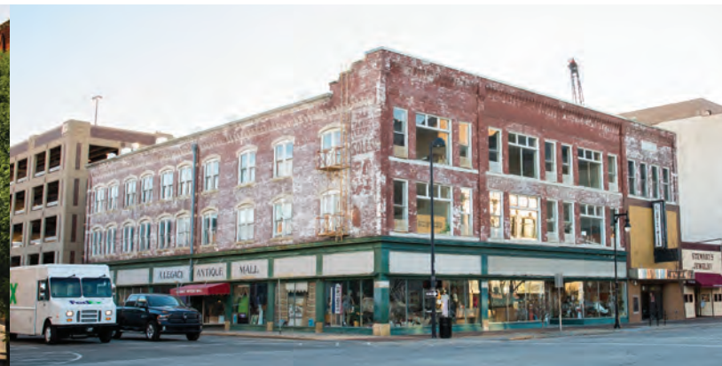
Douglas & Emporia Building Renovations N/A
