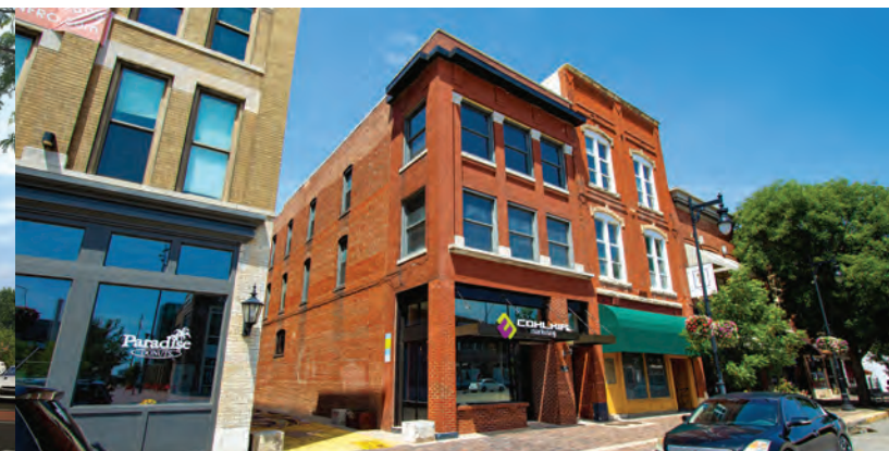
618 E. Douglas Avenue Renovations N/A
