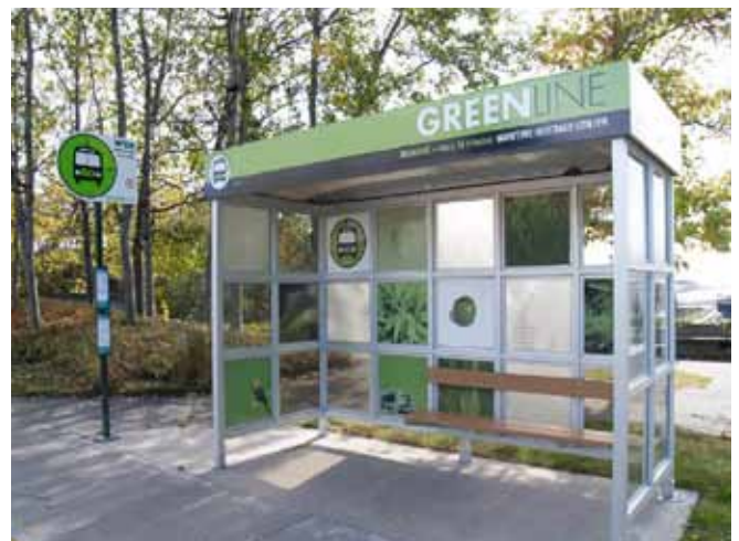
Transit Shelter with Integrated Signage
