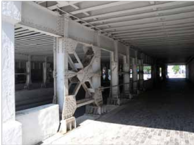
Existing sidewalk section beneath the BNSF corridor
