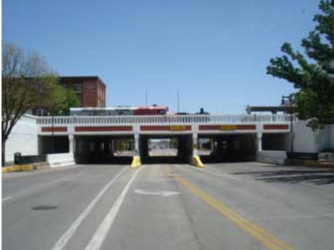
Existing rail viaduct
