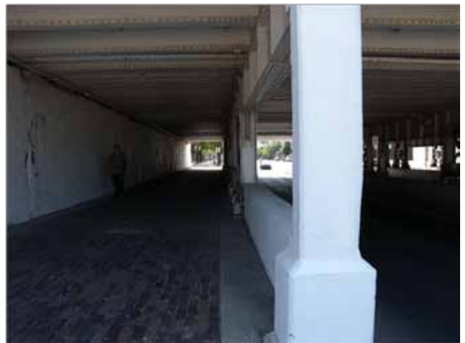
A pedestrian passes in the dark beneath the BNSF rail viaduct.
