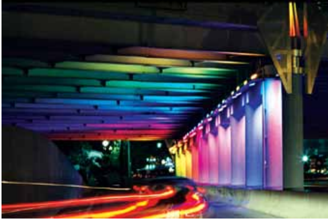
The Rossave underpass in Dallas, Texas
