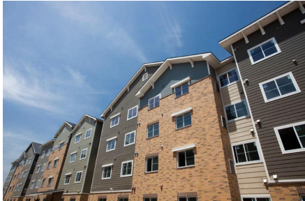
WaterWalk Hotel Apartments
