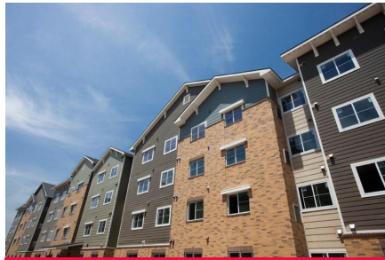
WaterWalk Hotel Apartments
