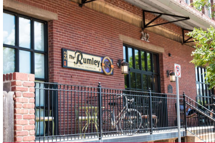
The Rumley Condominiums
