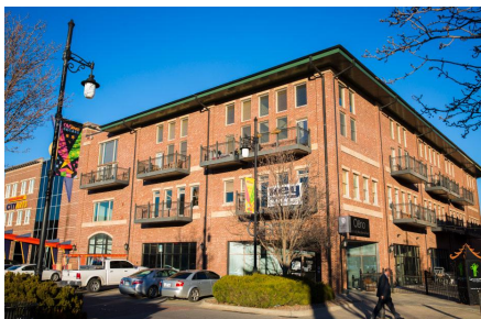
The Lofts at Old Town Square
