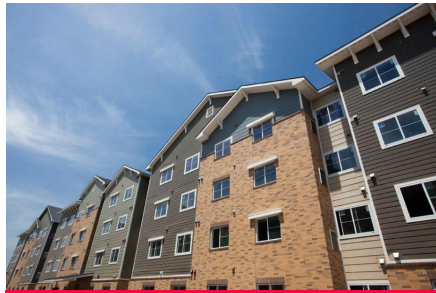
WaterWalk Hotel Apartments
