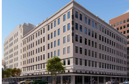
Former Innes Building into KHSC-KansasCom
