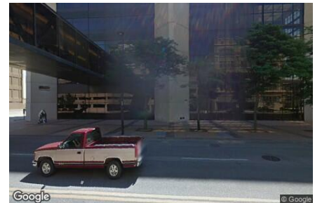
Petroleum Club of Wichita
