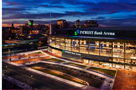
Cessna Plaza at INTRUST Bank Arena
