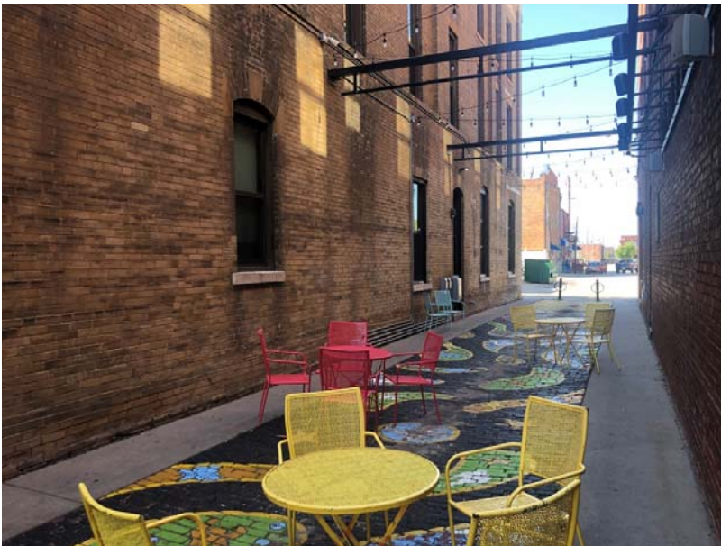
West wall, facing north.
