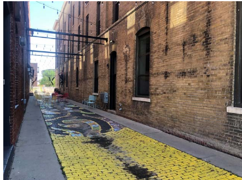
West wall, facing south.
