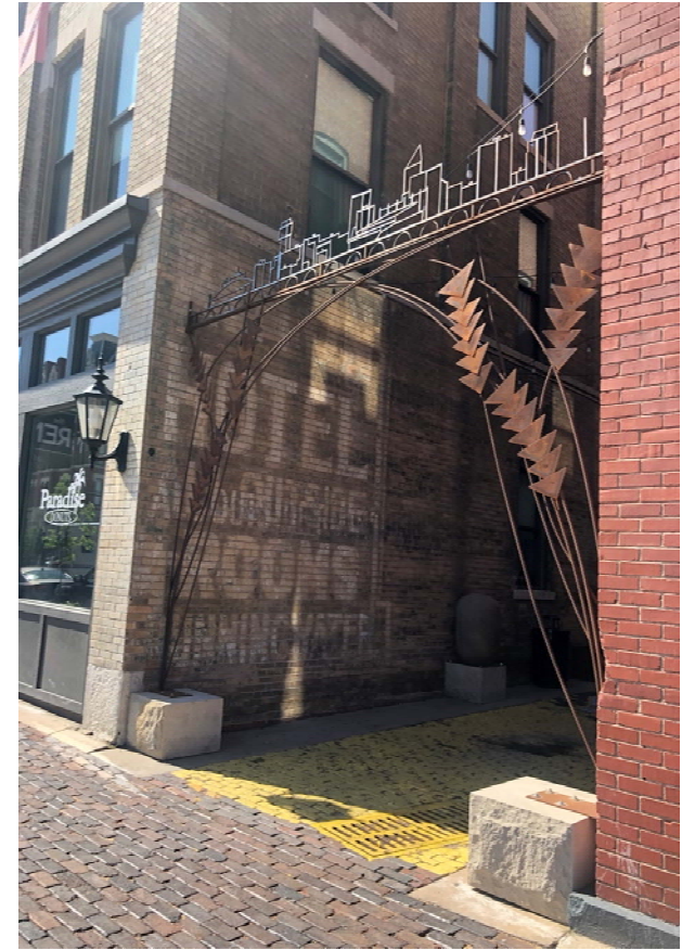
West wall, from Douglas Ave entrance
