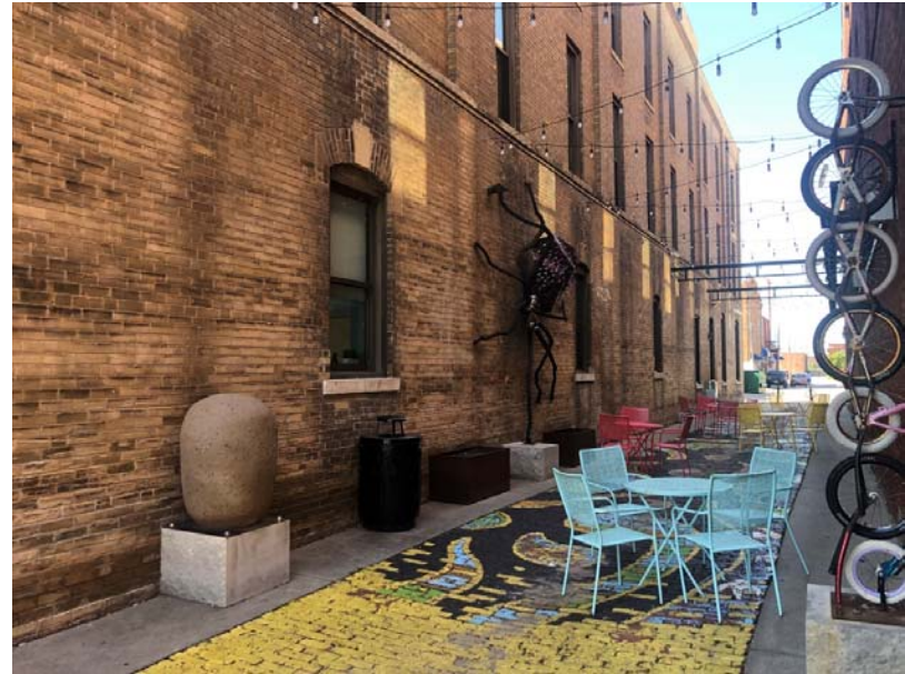
West wall, facing north.
