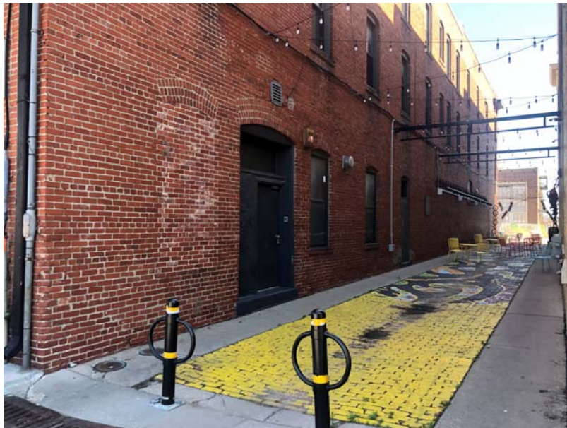
East wall, facing south, end of alley.
