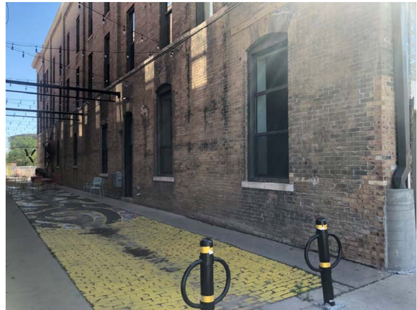
West wall, facing south, end of alley.
