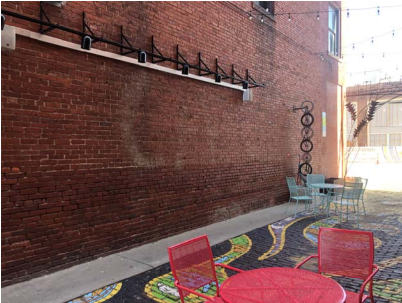
East wall, midway point facing south.
