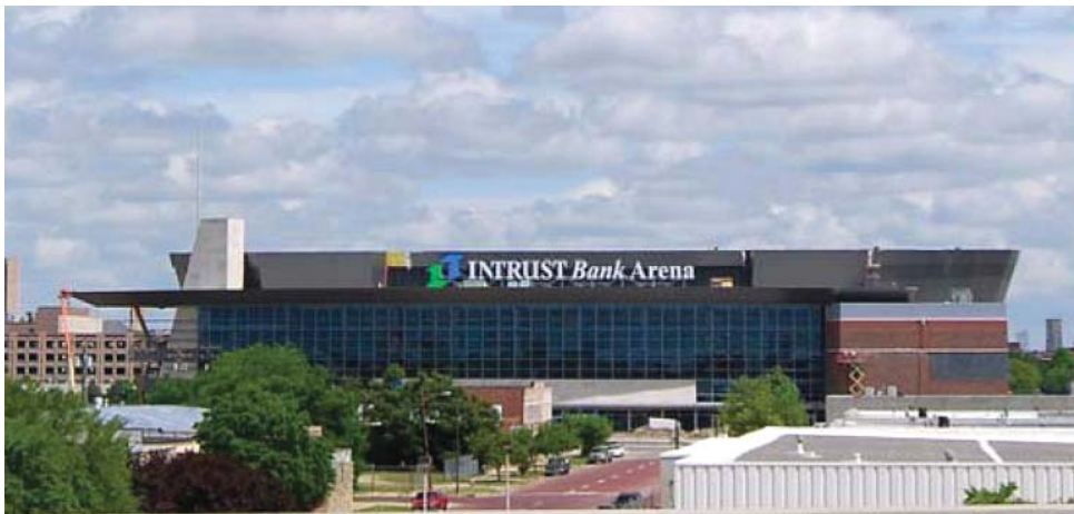
Intrust Bank Arena
