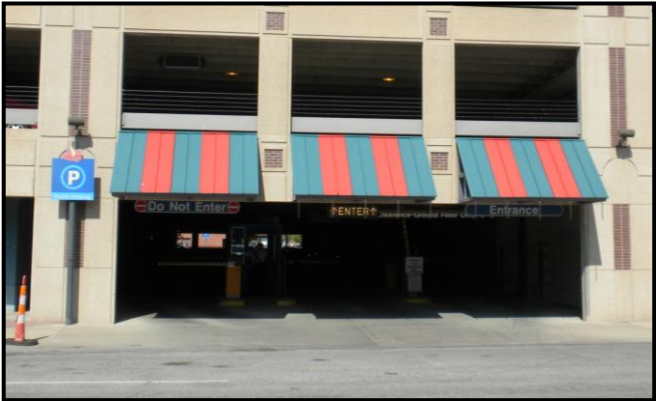
Current signage is installed parallel to the roadway, making it more difficult for drivers to see
