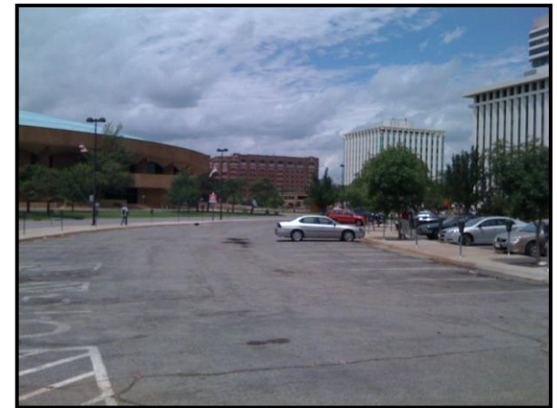
A thorough condition appraisal of public parking lots will determine maintenance needs/costs
