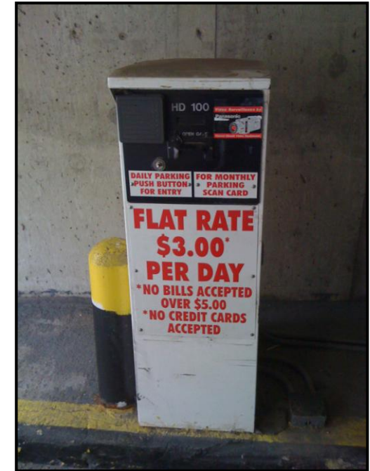
Quality revenue control requires parking access and revenue control equipment that is in good working condition
