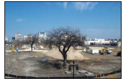
WaterWalk Construction Site, March 2007.
