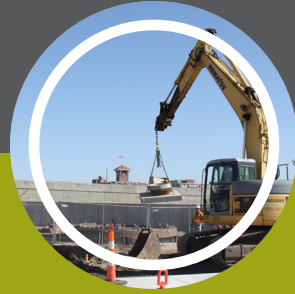
Construction on St. Francis
